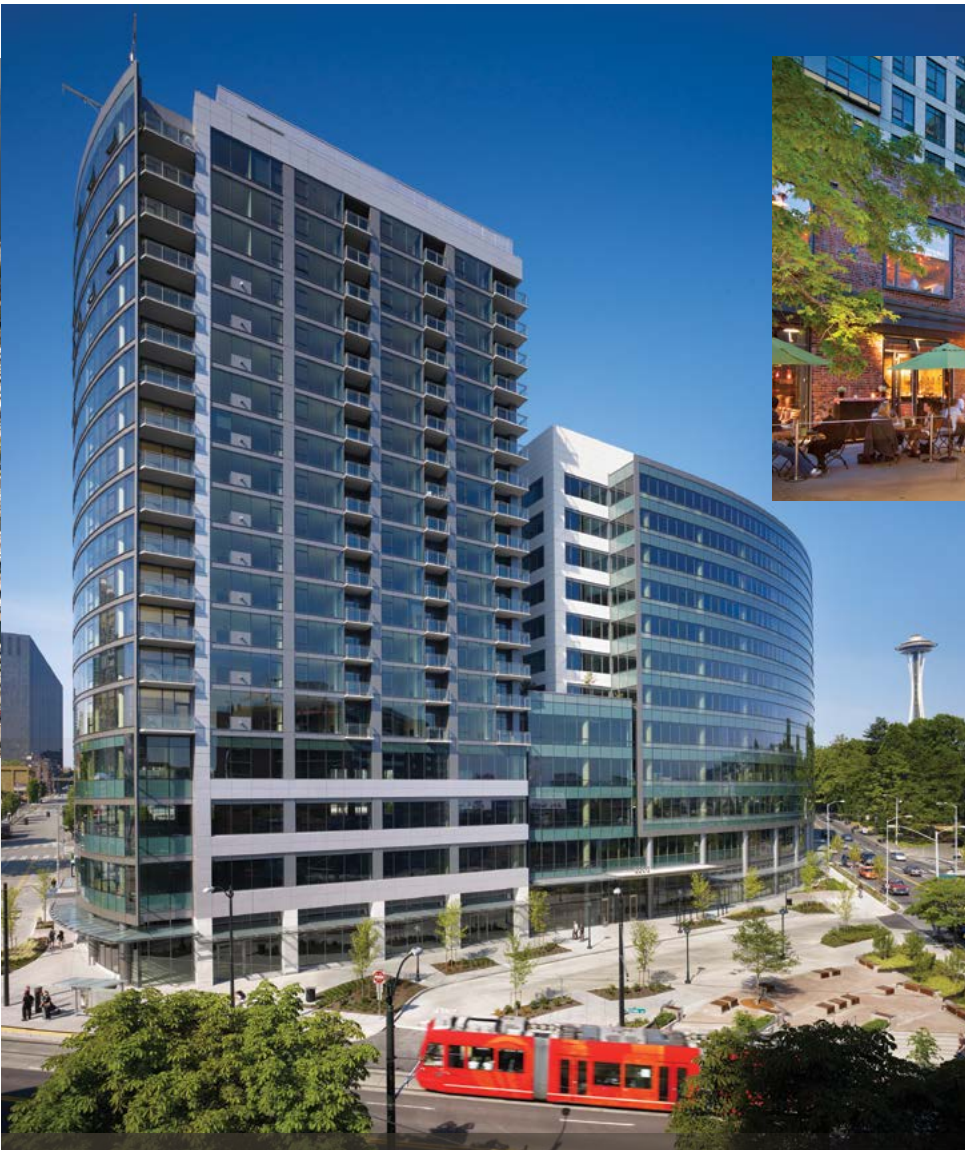
The 450,000-square-foot mixed-use LEED Gold 2201 Westlake building comprises a 12-story office tower and a 19-story residential condominium tower as well as retail space and subterranean parking.
